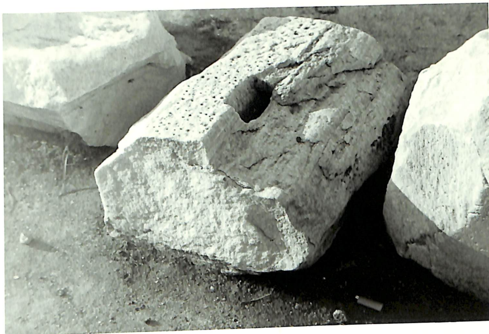
Figure 3a. Architrave Fragment with Broad Lewis Hole, Olympeion, Athens.
