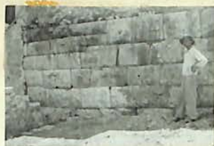
Fig. 13. Long wall on Pron, eastern stretch.
