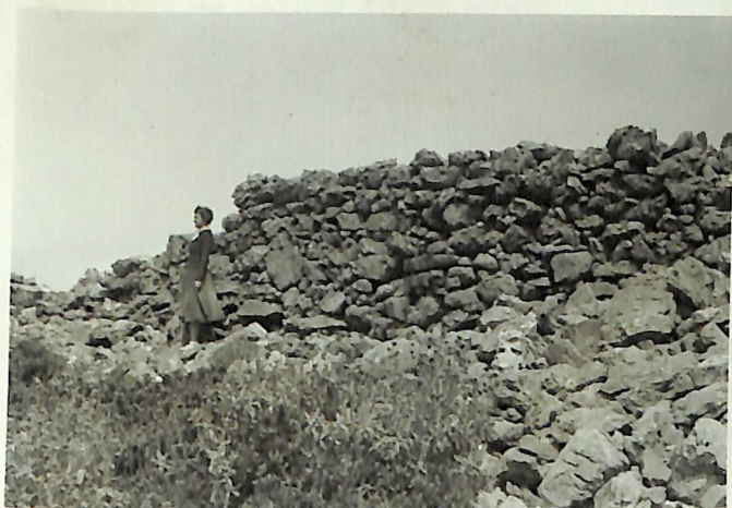
b. Koroni : West outer face of circuit wall
