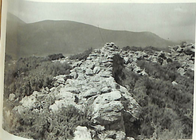
Koroni : top of circuit wall on NW side
