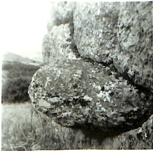
NEMEA BLOCKHOUSE - PROJECTION IN NORTH SIDE WITH SMALL WATER CHANNEL ON TOP.
