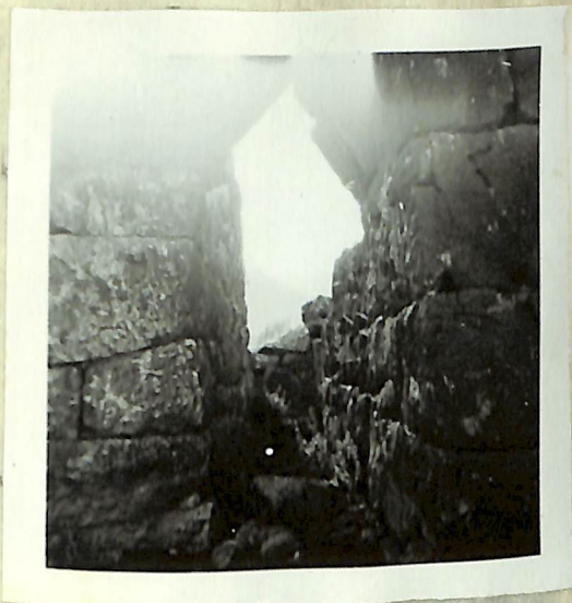
KEPHALARI PYRAMID - VIEW FROM E. OF DOORWAY (AT S. END OF E. SIDE) NOTE TRIANGULAR OPENING AT TOP.
