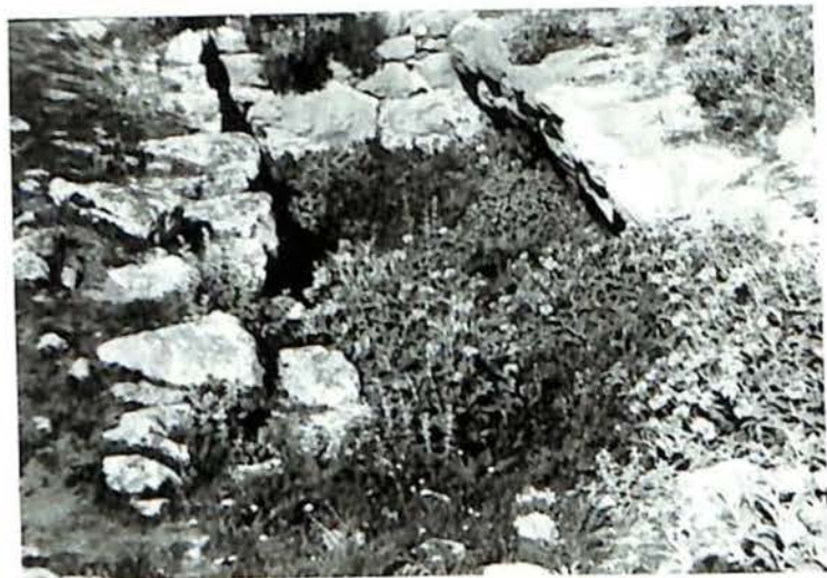
Fig.19. Kasarma, View of the Water Cistern.
