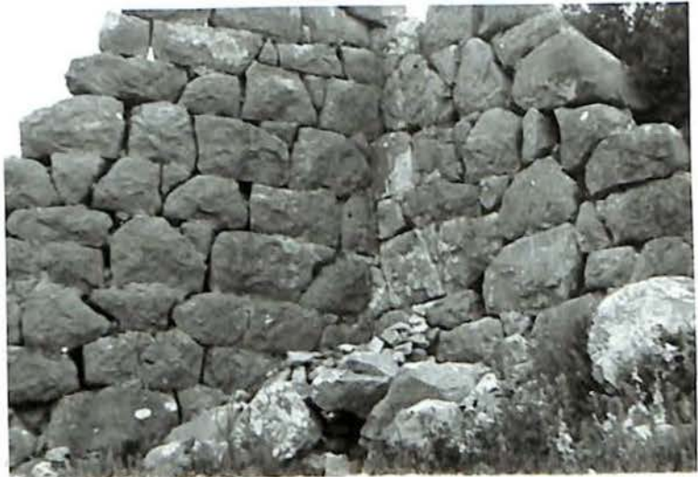
Fig.25. Kastraki, Bonding of Curtain and Gate Tower.
