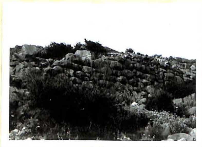
Fig.8. Kasarma, the Ramp Wall from below.
