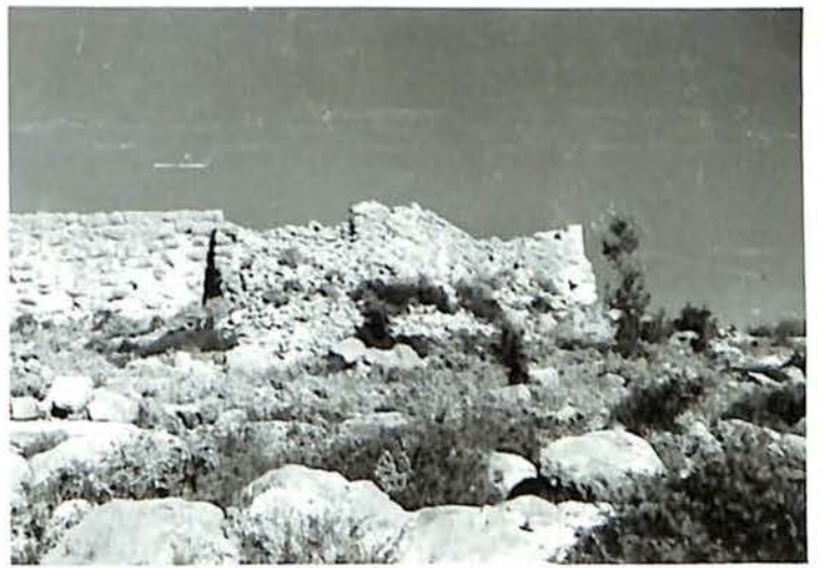
Fig.16. Kasarma, Tower III and the Adjoining Curtains.
